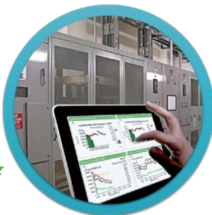
Power Quality Monitoring
